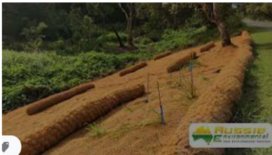
Coir logs and coco logs wrapped with coir netting for a sloppy terrain
